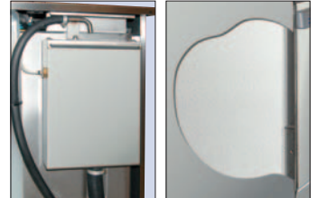
WRAS approved category 4 integral break tank and washtank insulation.
