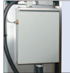
WRAS approved category 4 break tank c/w integral rinse booster pump.
